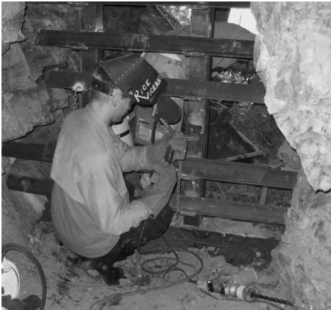
Welder John Norman completes a steel bat gate enclosure
