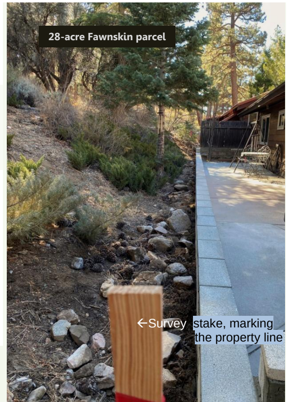
This 2-ft wall was dismantled and rebuilt in-bounds
